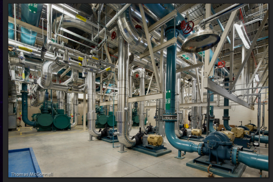
TACC Machine Room Chilled Water Plant
